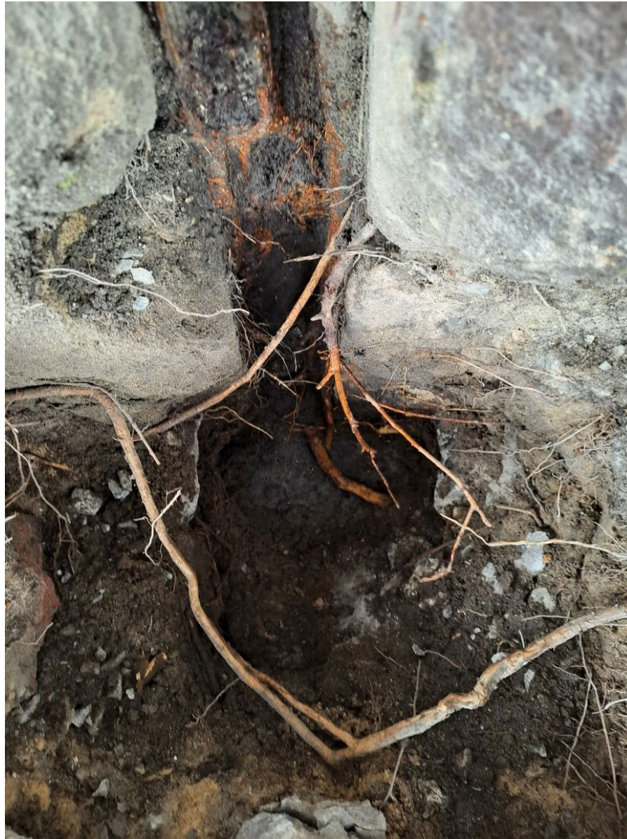
Photo A: Roots from Tree 1 shown growing under the footpath, but partially impeded by the existing Sewer encasement which is to be demolished as part of the development.
